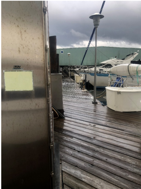
Photo 4. N Dock Open Timber Float
