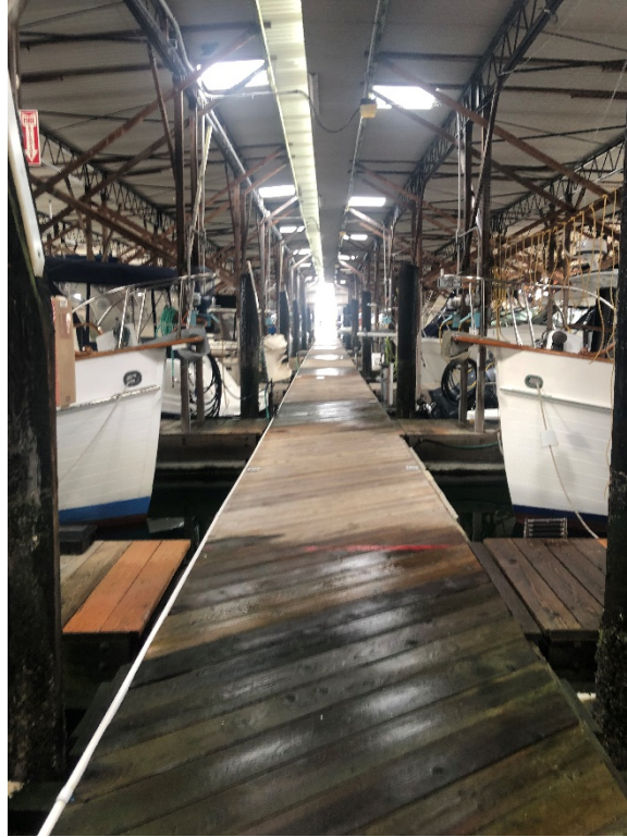
Photo 7. Covered Moorage System
