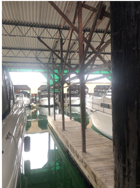
Photo 6. Timber Framing and Roof Structure
