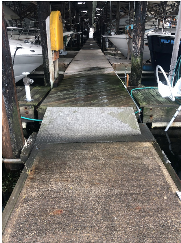
Photo 14. Transition from Timber to Concrete Dock
