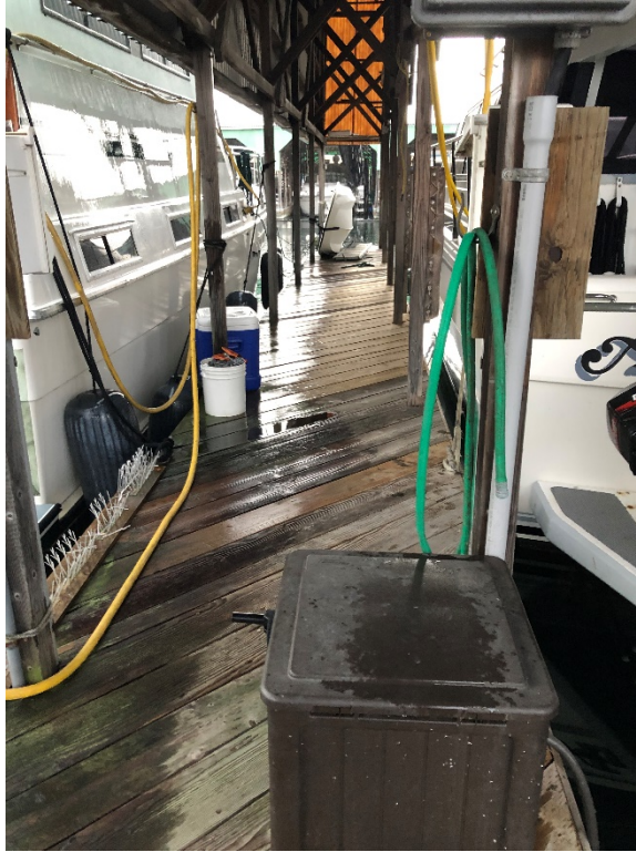
Photo 3. N Dock Timber Finger
