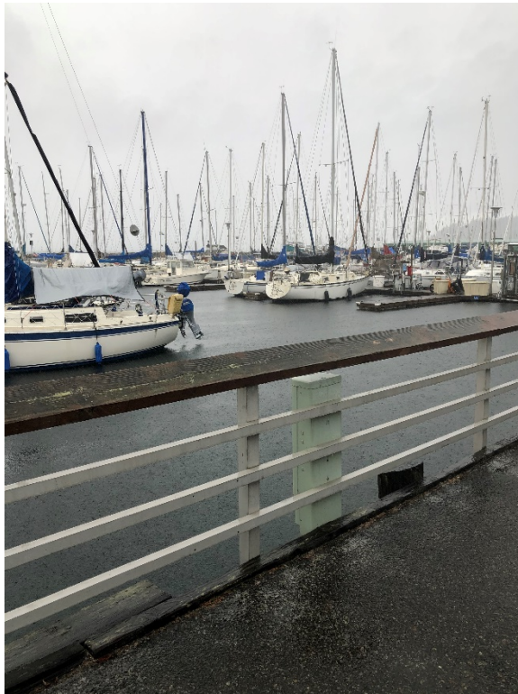
Photo 20. A and B Concrete Docks
