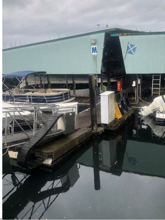
Photo 5. M Dock Roof Structure
