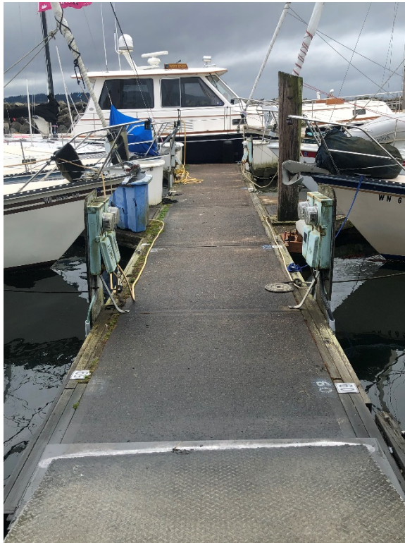
Photo 10. Outer Uncovered Concrete Dock System
