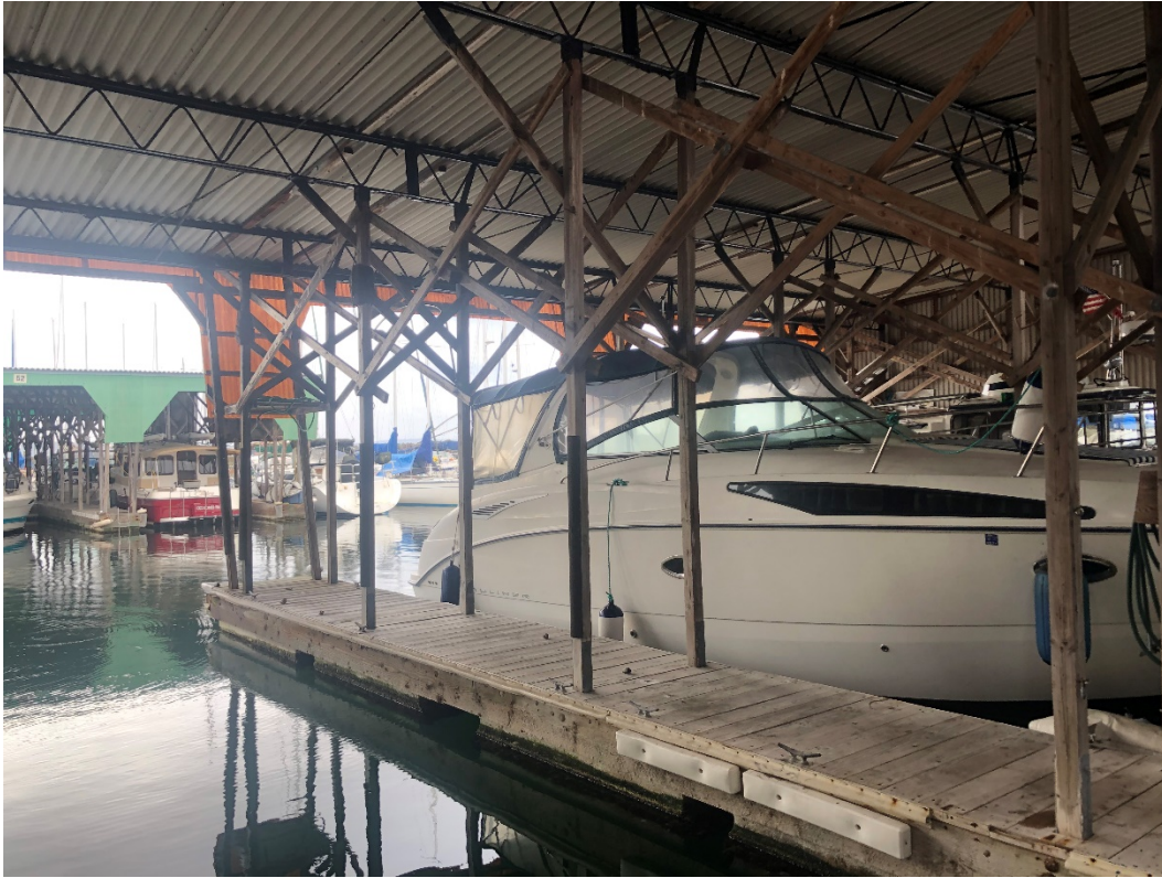
Photo 13. Covered Moorage System Timber Float
