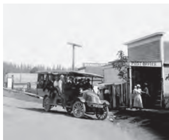
Early transit in 1914. Note wooden sidewalk. This is east side of 6th Avenue, between 223rd and 225th.
