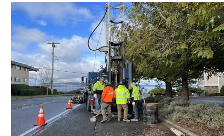
Geotechnical boring along South 223rd Street
