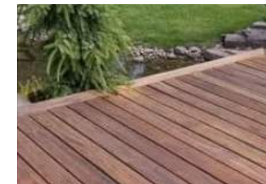
Deck seating area over bioswale
