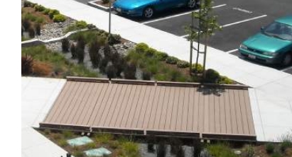
Pedestrian bridge over bioswale
