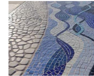
Decorative mosaic crosswalk treatment
