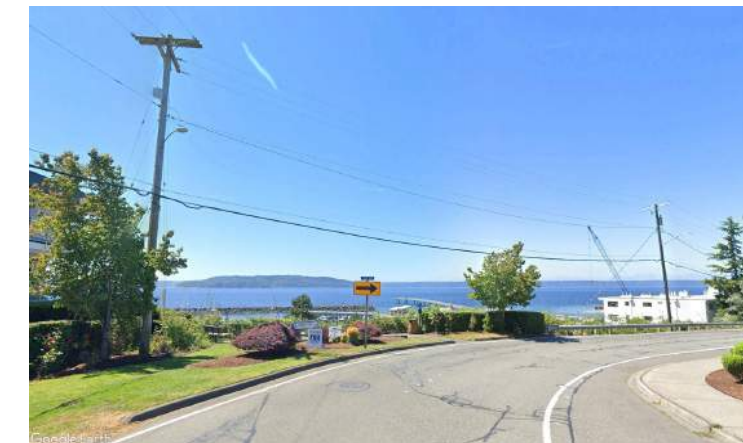
Overhead utility lines at Overlook I Park
