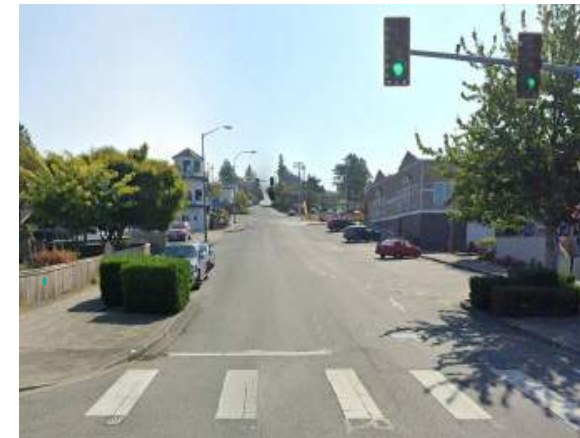
Looking east up S. 223rd St. from 7th Ave S.
