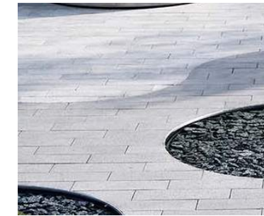
Decorative cement paver treatment
