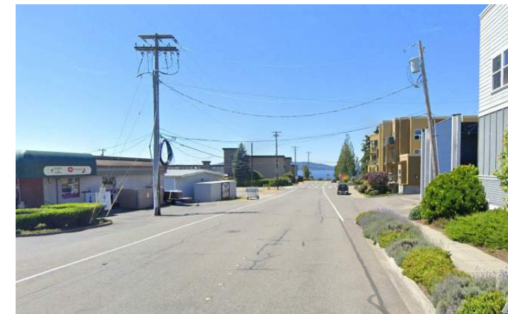
Overhead utility lines just east of S 223rd St and 7th Ave S intersection
