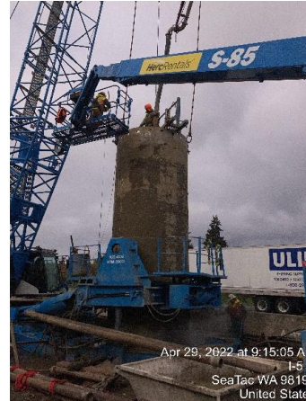
NBCD Bridge Pier 3 Shaft, SeaTac
