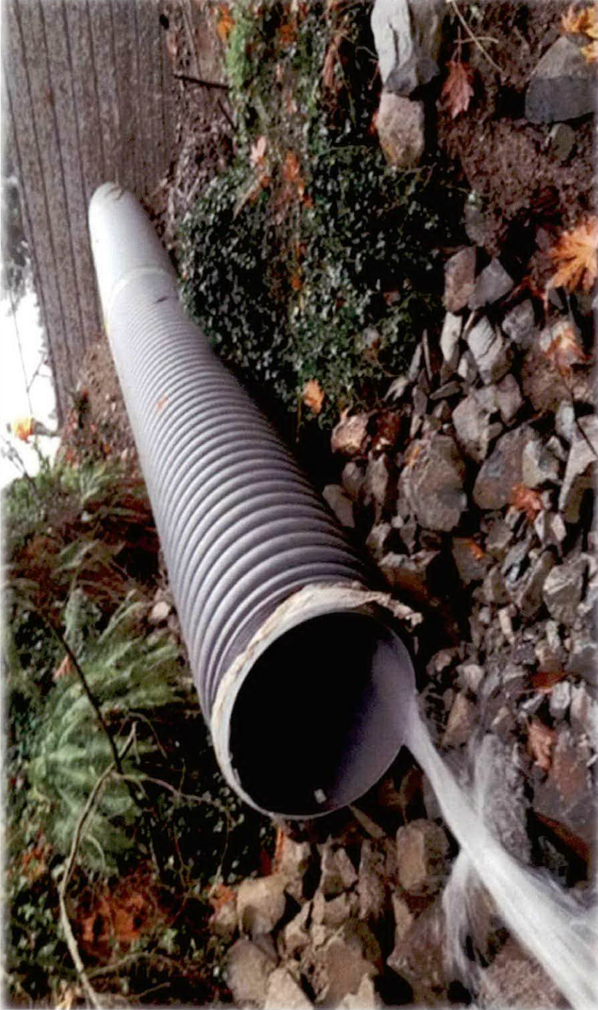
S. 251st Street Storm Outfall
