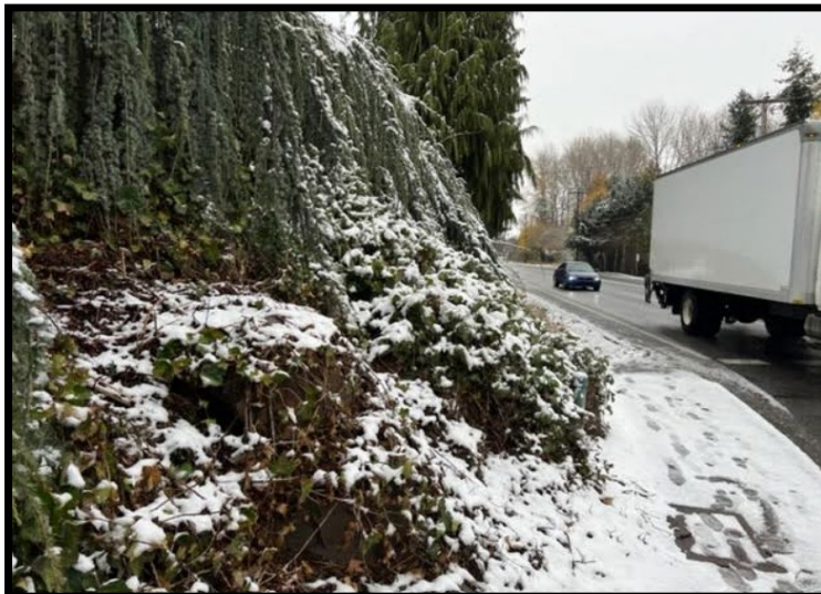
Facing East Along the Subject's S. Kent-Des Moines Road Frontage.
