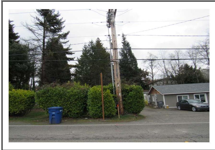
Photograph of the power pole to be removed and relocated.
