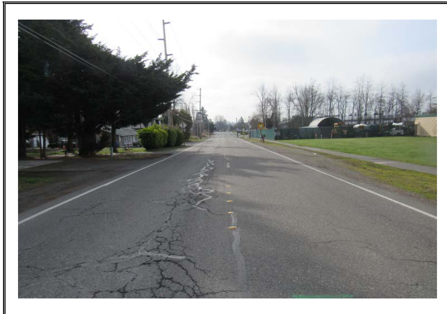
Access to the subject property facing north from 24 th Avenue South.
