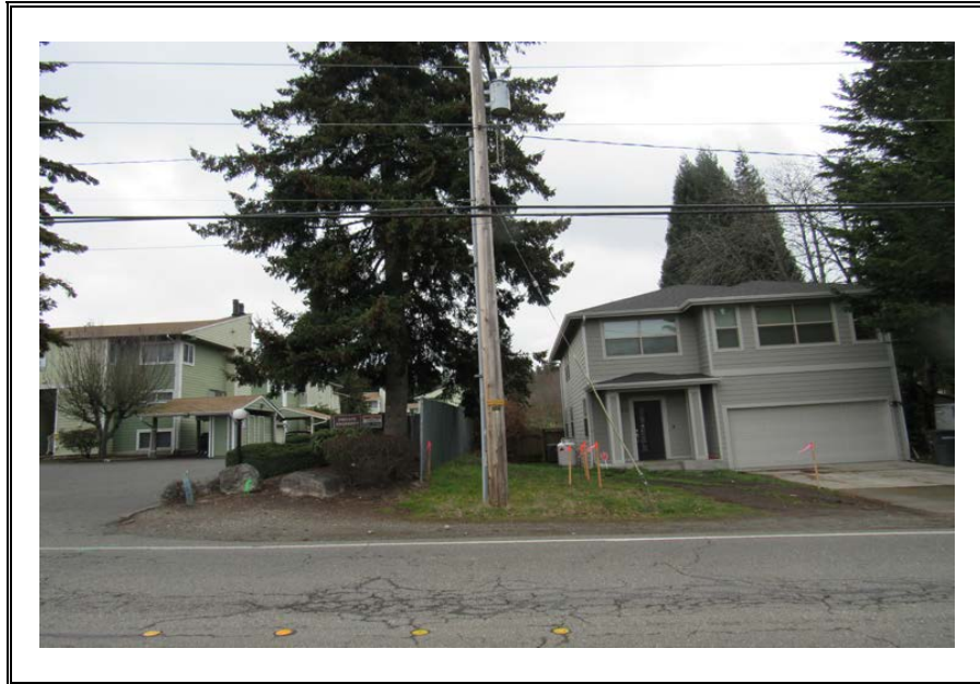
Photograph of the power pole to be moved and relocated.
