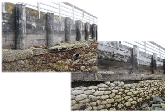
Figure 2-13. Old North & West Timber Pile Bulkhead
