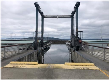
Figure 2-9. Travel Lift Pier
