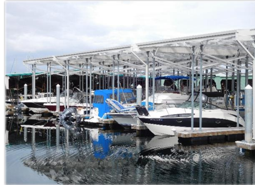
Figure 4-2. Covered Moorage on J-Dock
