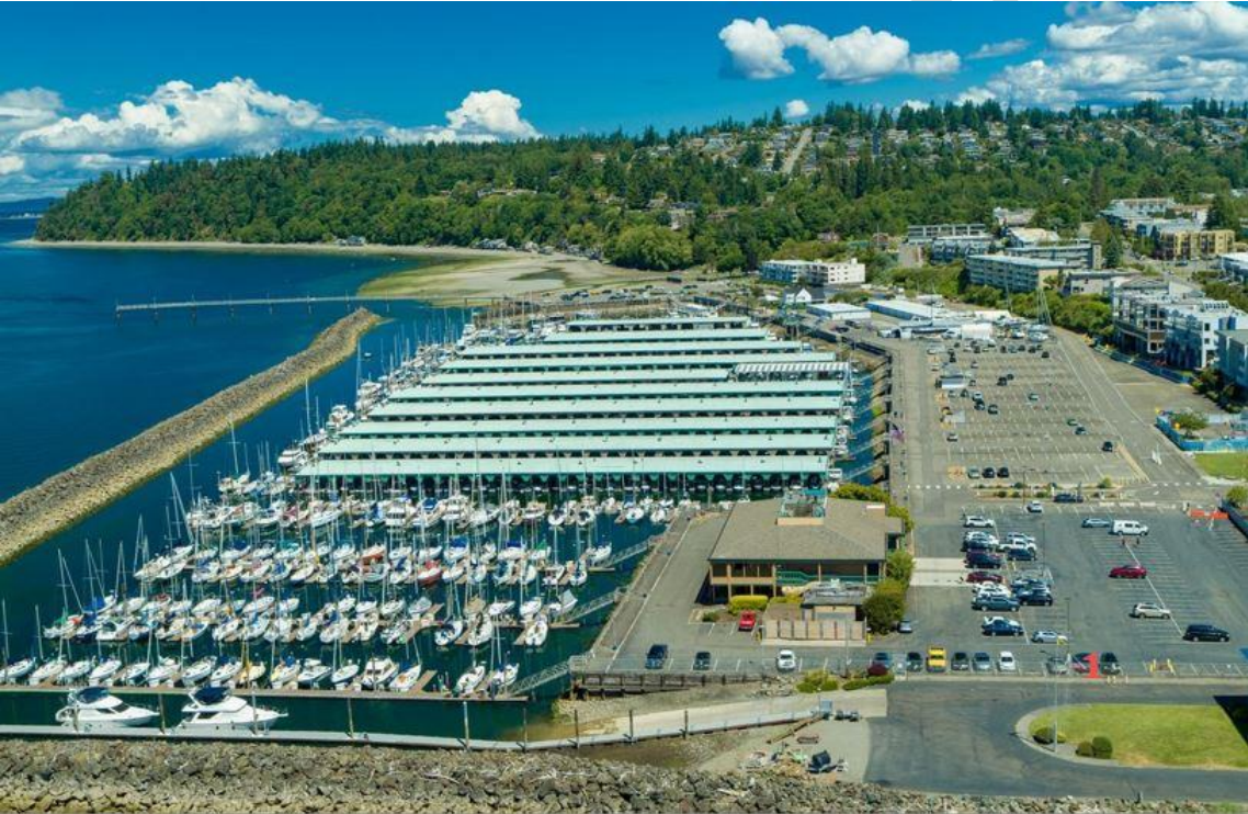
Figure 1. City of Des Moines Marina
