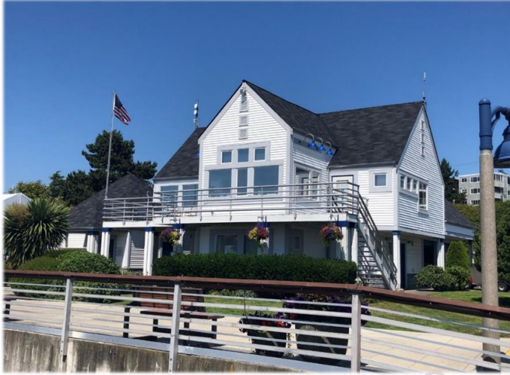
Figure 5-1. Marina Office Building July 2021
