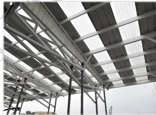
Figure 4-3. Light-Penetrating Covered Moorage
