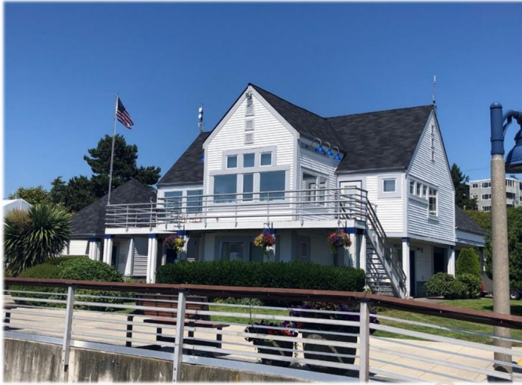
Figure 5-1. Marina Office Building July 2021
