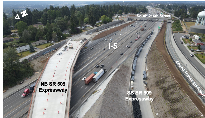
I-5 looking south
