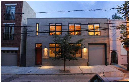
Philadelphia, PA Contractor shop converted to 3 bedroom house with large office space
