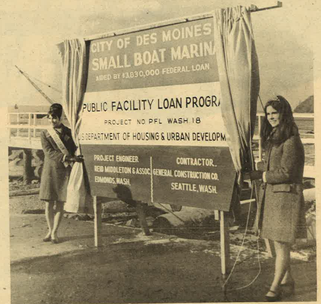
MISS BOAT SHOW, left, and Miss Des Moines 1969, Sue Shaffer, unveil construction sign at rock dropping ceremony January 21, 1969.
