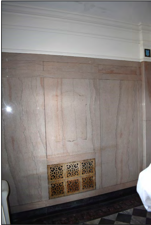
Fig. 46 – Main Building, interior, first floor, entry vestibule.
