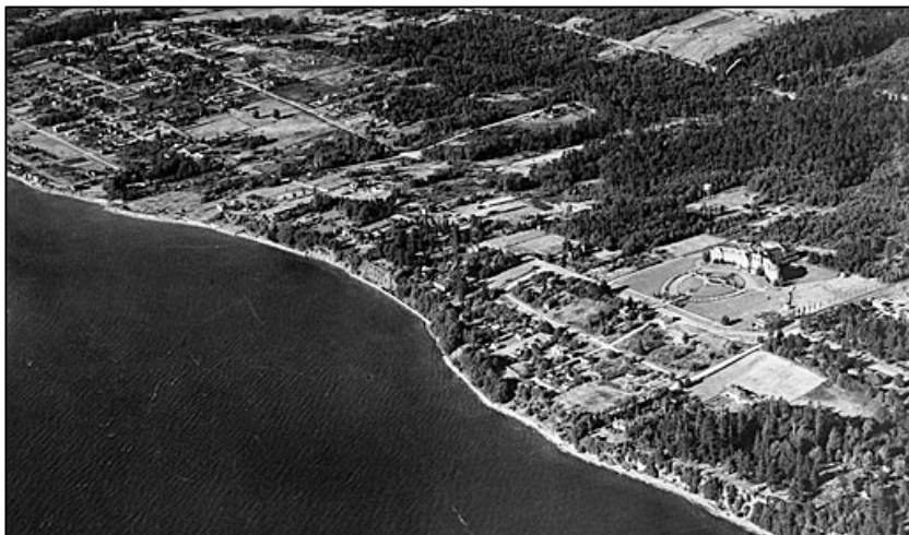
Des Moines and Zenith around 1935. Until the 1950s, most of the development in this area was largely confined to a strip of land a few blocks deep, along the waterfront. The Masonic Home at lower right was the most imposing structure in the vicinity. (Washington Historical Society 2004.0.963)
