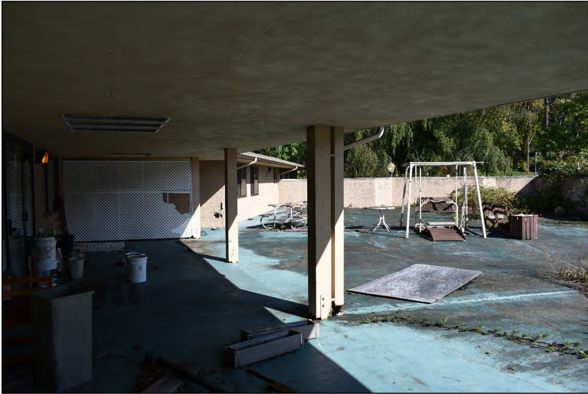
Fig. 28 – Infirmary Wing, outdoor walled exercise area, view east from building.
