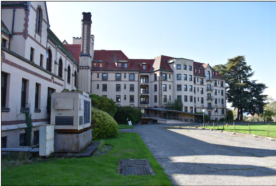
Fig. 13 – Main building, view west to east and north elevations.
