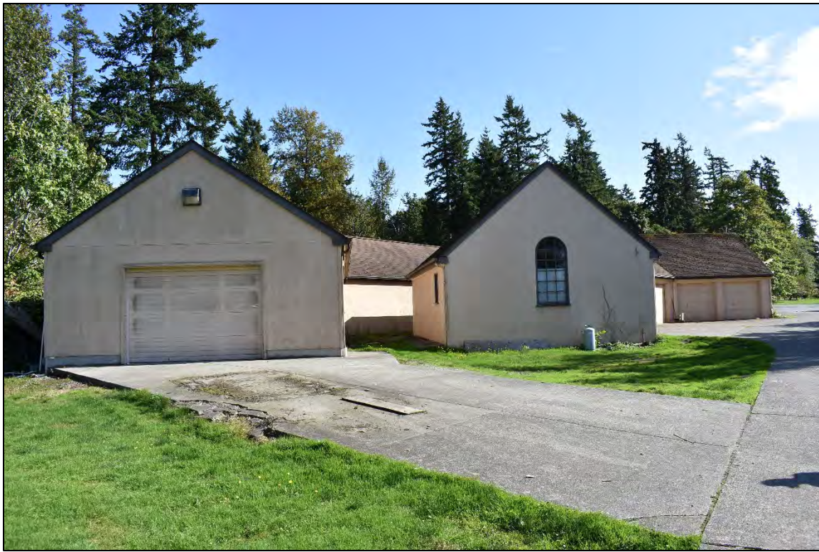
Fig. 39 – Storage Building at left (built 1997); Garage at right (built 1937).
