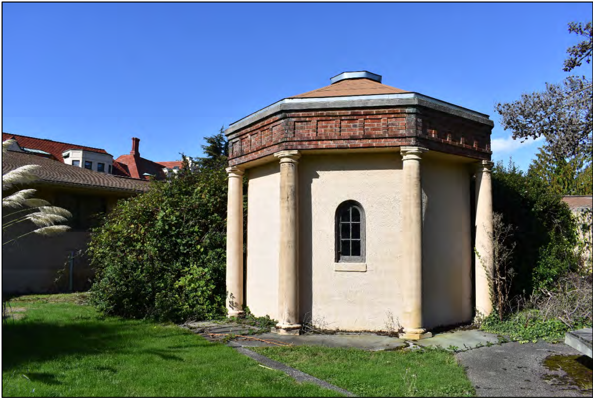
Fig. 26 – Octagonal Pumphouse, south elevation.
