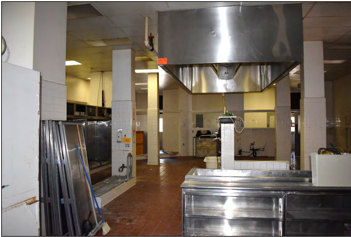
Fig. 57 – Main Building, interior, first floor, kitchen.
