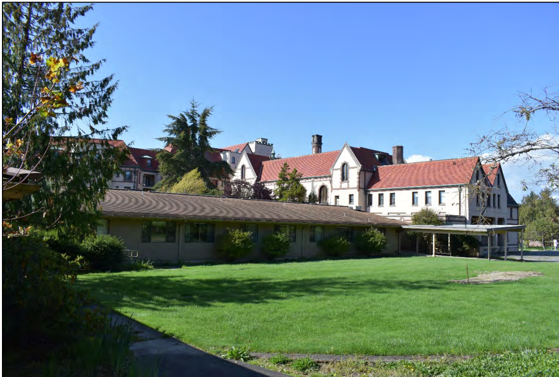
Fig. 20 – Infirmary Wing, east elevation of north arm, view to northwest, with Main Building rear wing south elevation.
