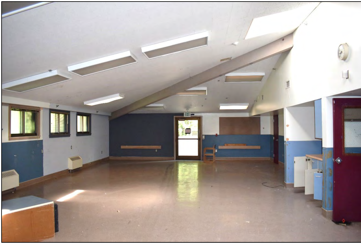
Fig. 95 – Infirmary Wing, interior, first floor, east arm (built 1987), view east.
