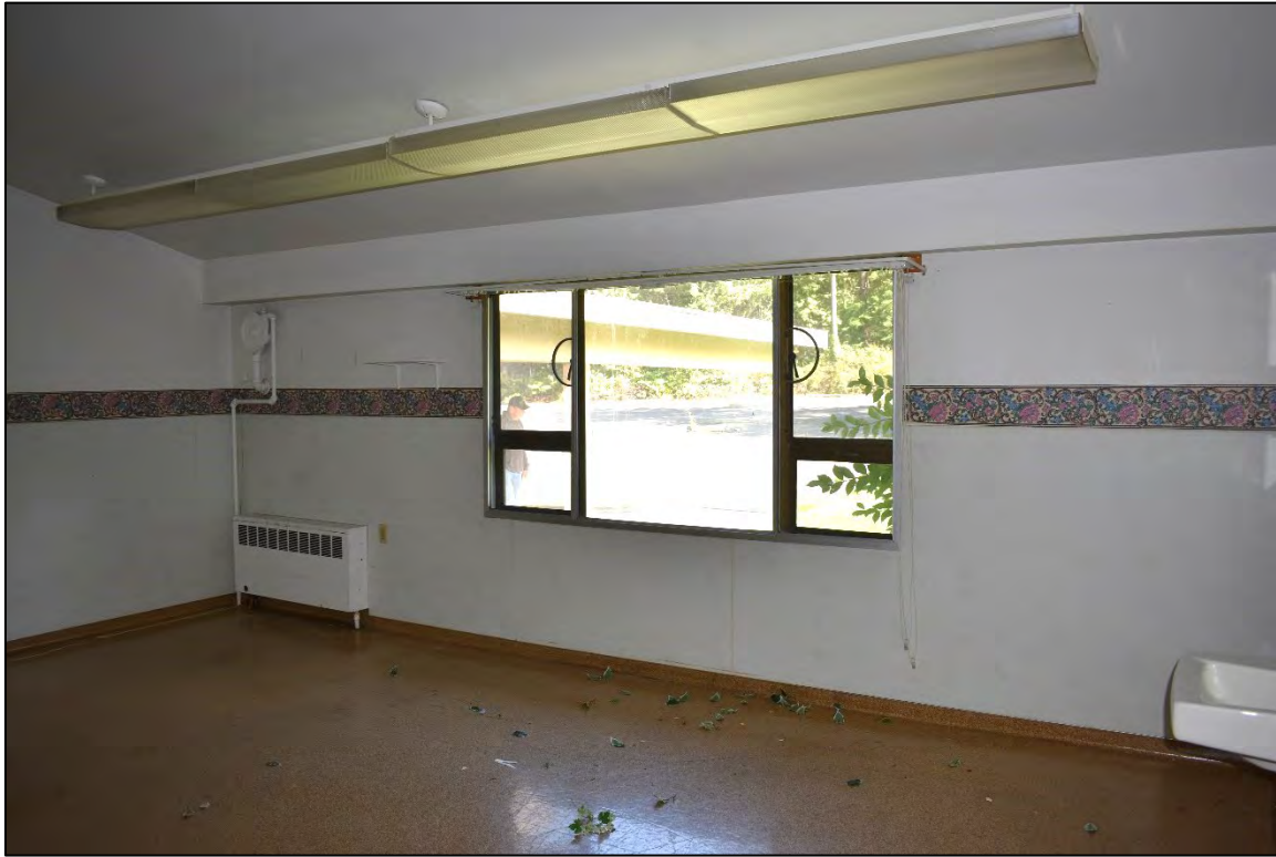
Fig. 92 – Infirmary Wing, interior, first floor, typical ward along corridor (built 1966).
