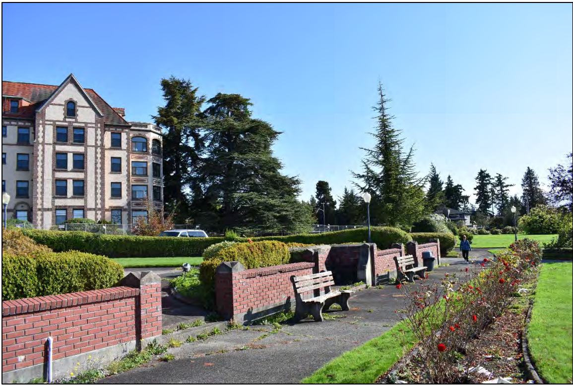
Fig. 37 – Central Oval, brick retaining wall at walk, view south.
