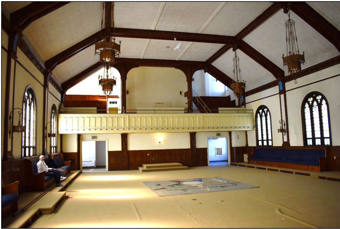
Fig. 65 – Main Building, interior, second floor, chapel/auditorium, view west to rear.
