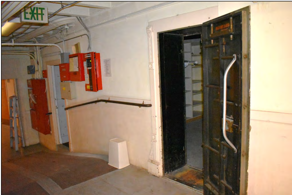
Fig. 88 – Main Building, interior, basement, corridor at vault room.
