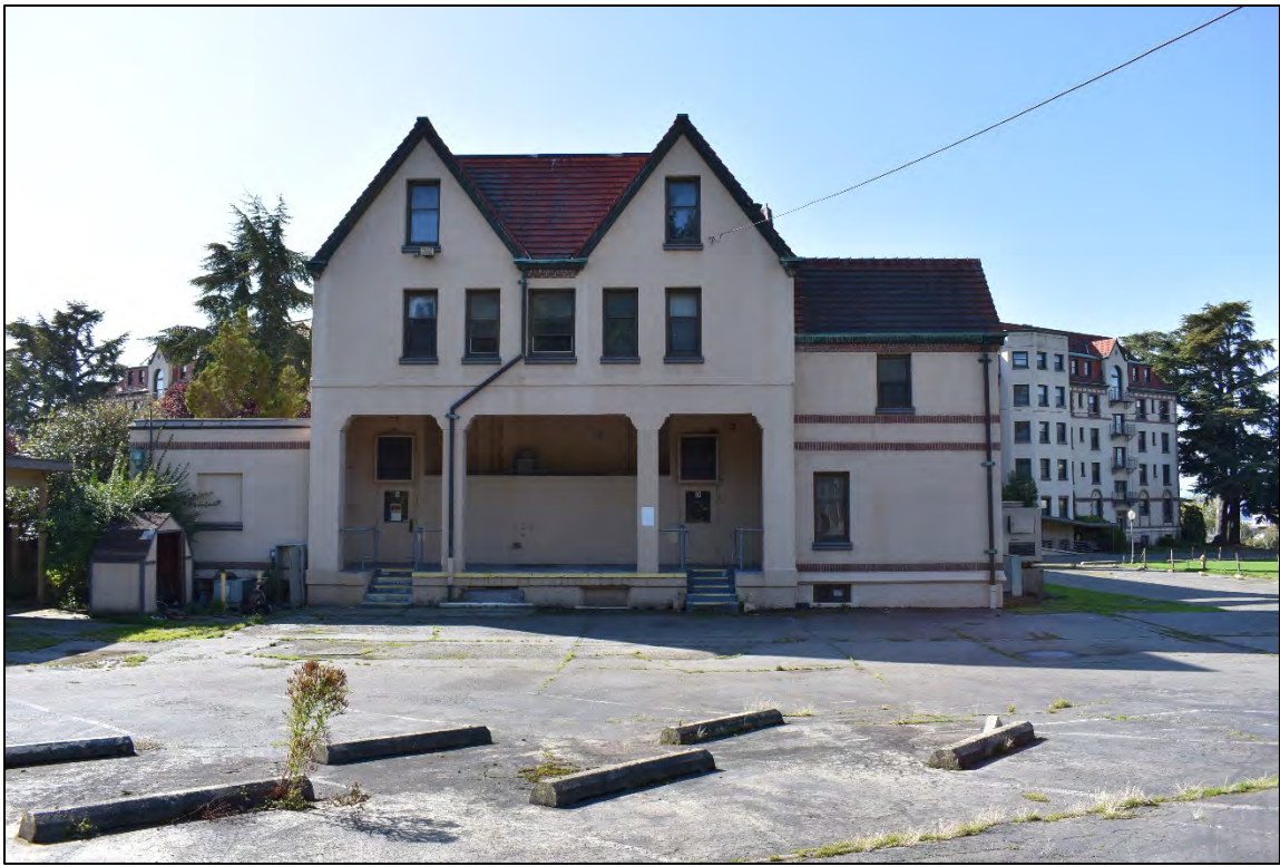
Fig. 15 – Main building, east elevation, rear service wing, showing loading dock.
