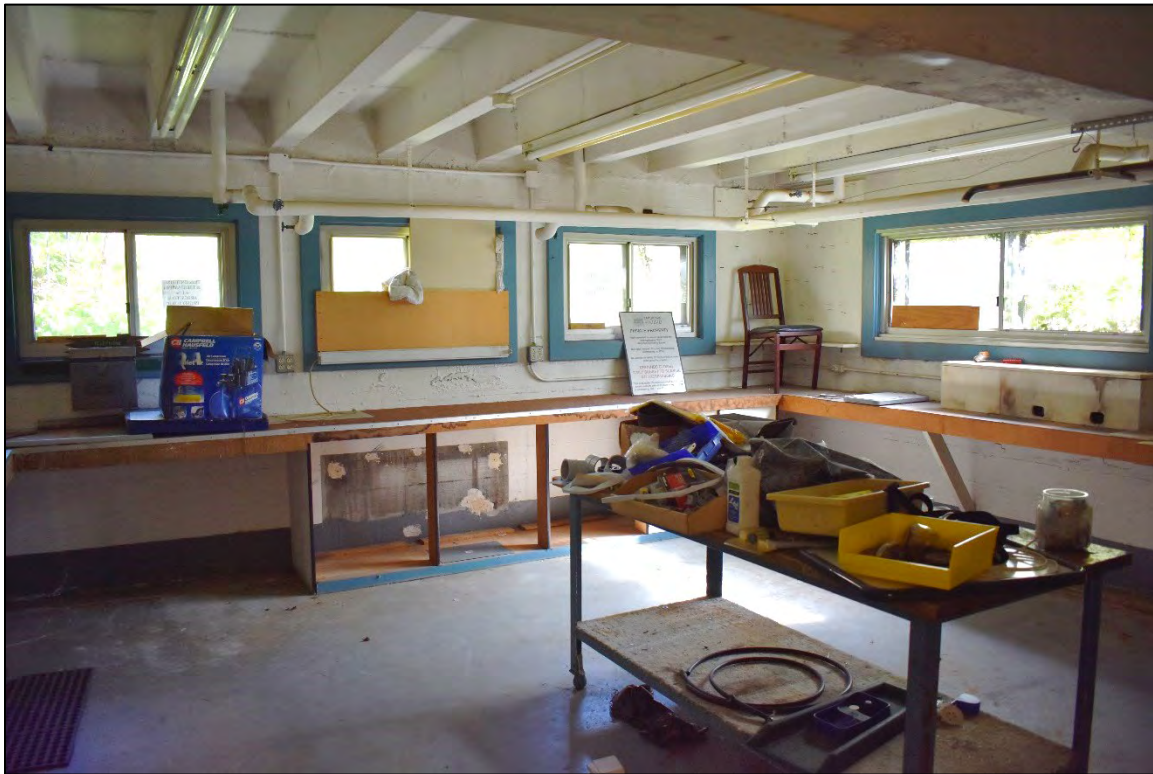
Fig. 90 – Main Building, interior, basement, typical room, showing concrete floor structure overhead.
