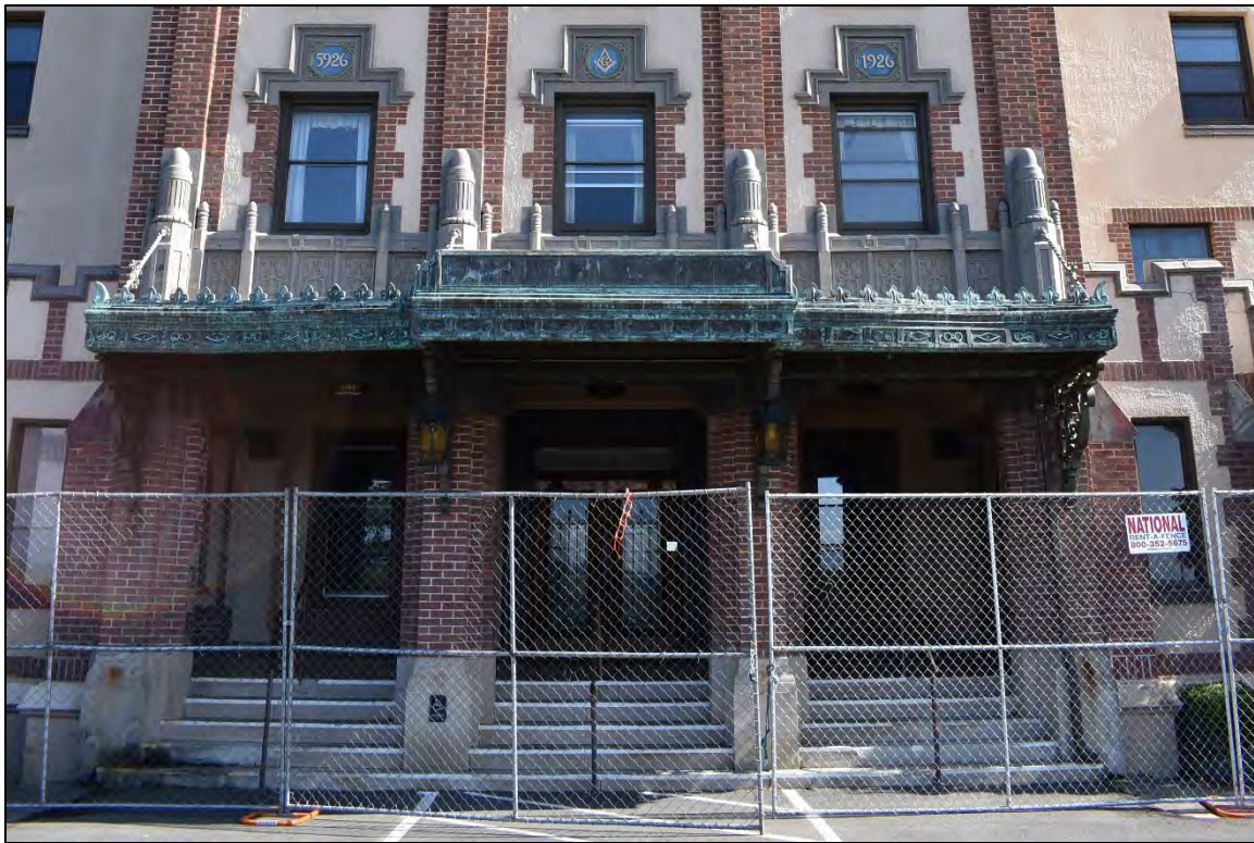
Fig. 45 – Main Building, front entrance.
