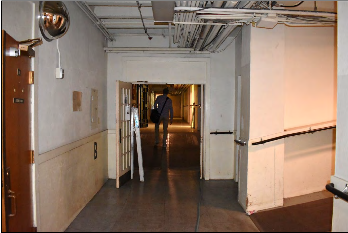
Fig. 86 – Main Building, interior, basement, typical corridor.
