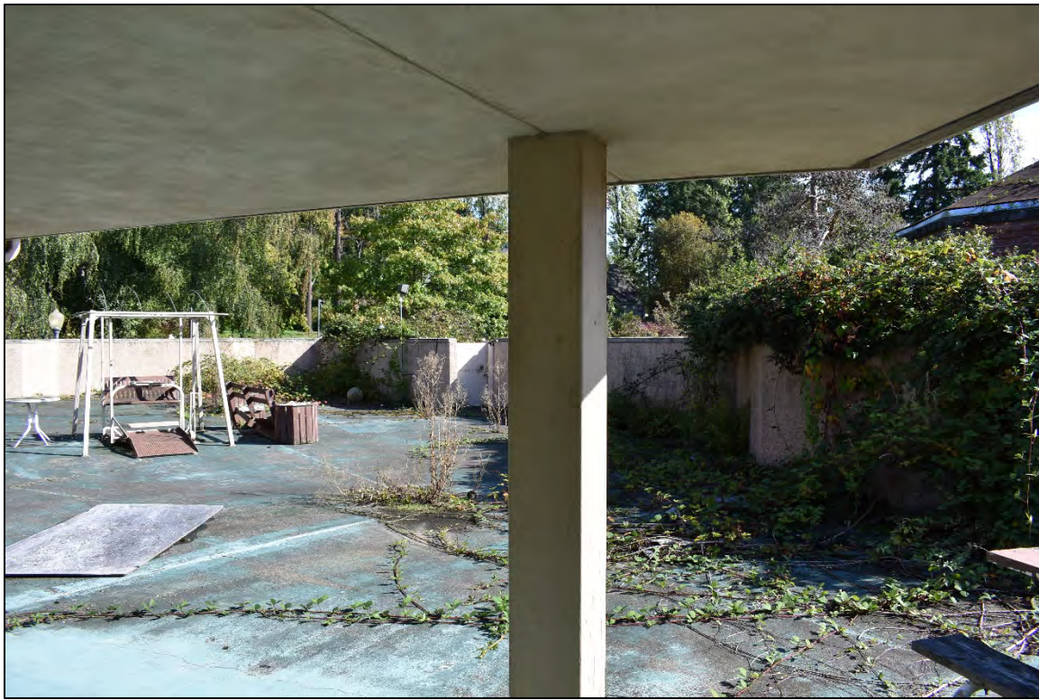
Fig. 29 – Infirmary Wing, outdoor walled exercise area, view south from building.
