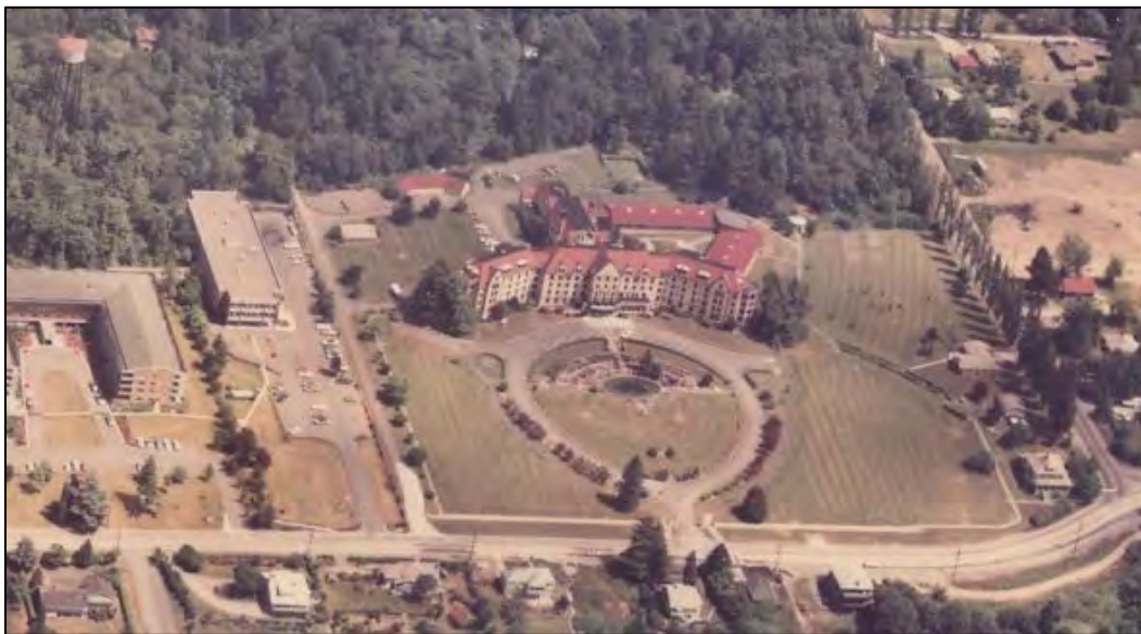
Masonic Home in 1977, showing 1966 Infirmary Wing at rear, which would be expanded in 1987. North is oriented left.
