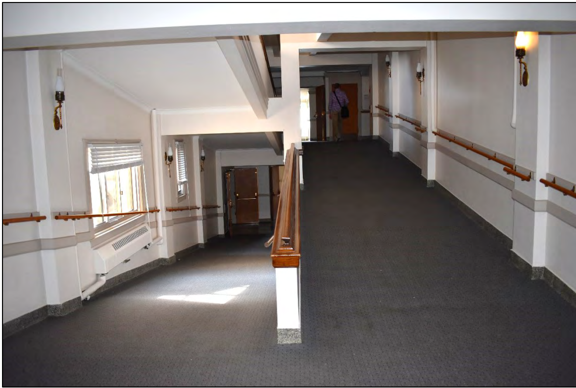
Fig. 61 – Main Building, interior, upper floor, main circulation ramps, longitudinal view.
