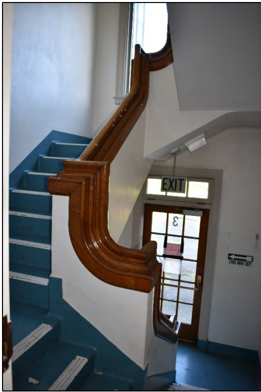
Fig. 63 – Main Building, interior, typical secondary stair.
