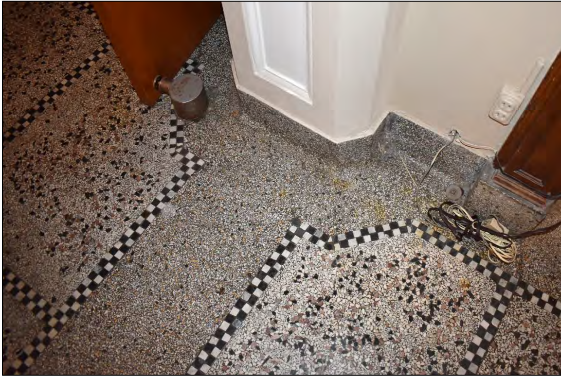
Fig. 48 – Main Building, interior, first floor, main hall, detail of terrazzo floor.
