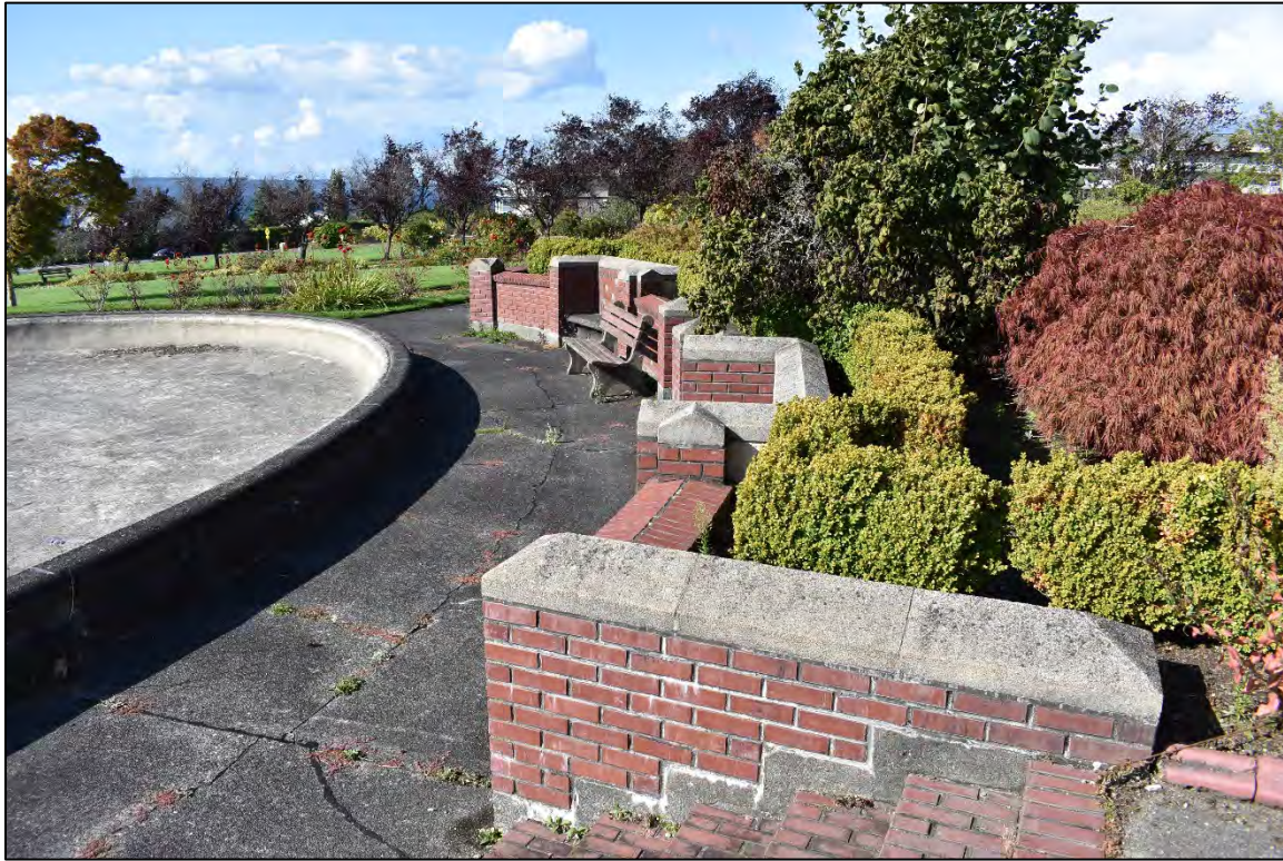
Fig. 36 – Central Oval, curved brick retaining wall at pool, view north.
