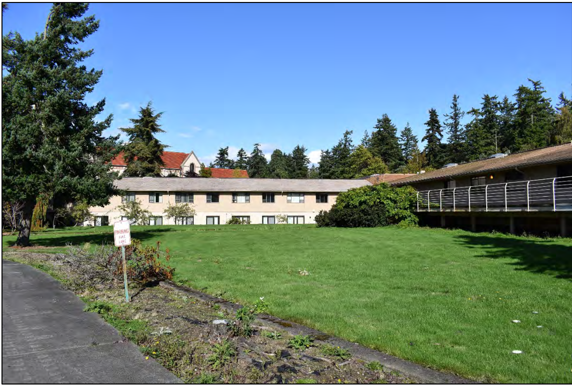
Fig. 33 – Infirmery Wing, view north from west yard, showing northwest arm (1966) at left and southwest arm (1987) at right.
