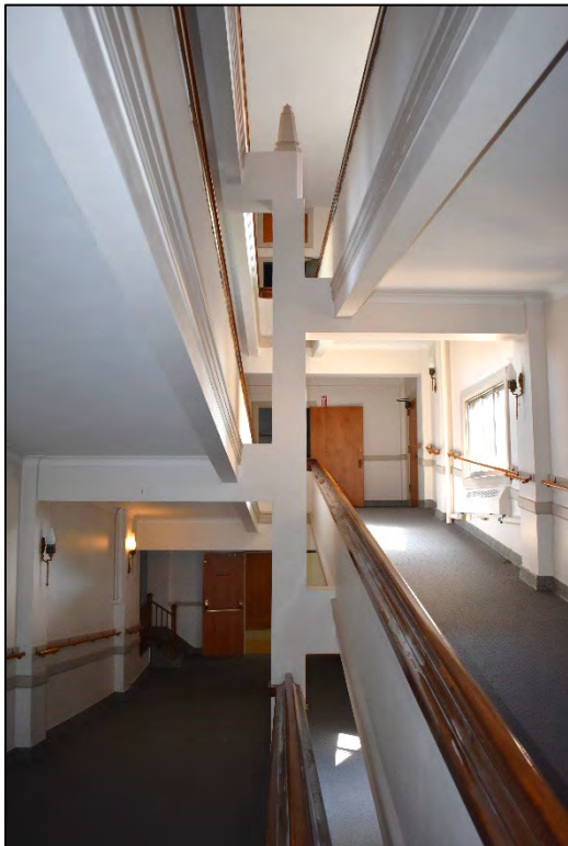
Fig. 62 – Main Building, interior, upper floor, main circulation ramps, longitudinal view and support column.
