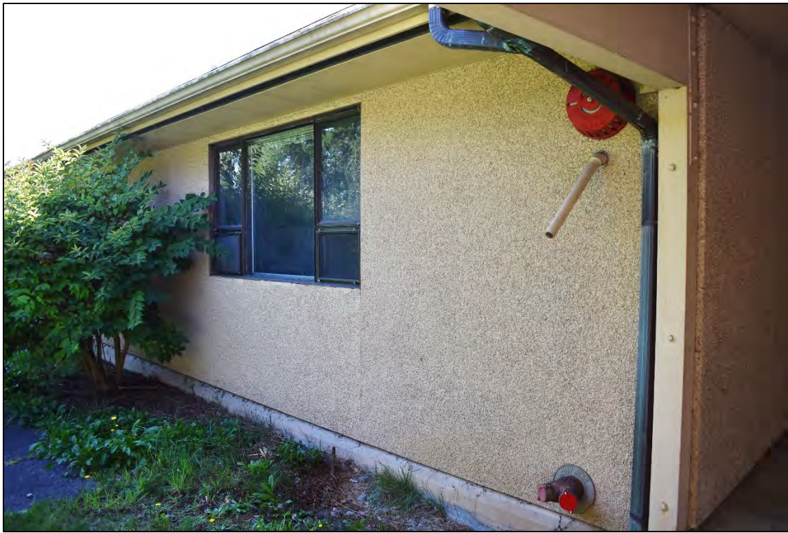
Fig. 21 – Infirmary Wing, east elevation of north arm, detail of marblecrete wall.
