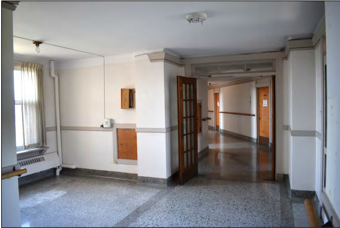
Fig. 76 – Main Building, interior, upper floor, typical residential wing mid-corridor sitting area.
