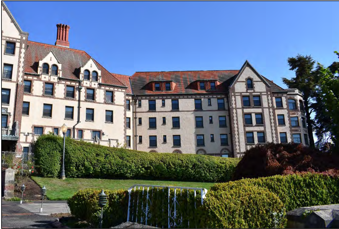
Fig. 4 – Main building, west elevation, south wing.
