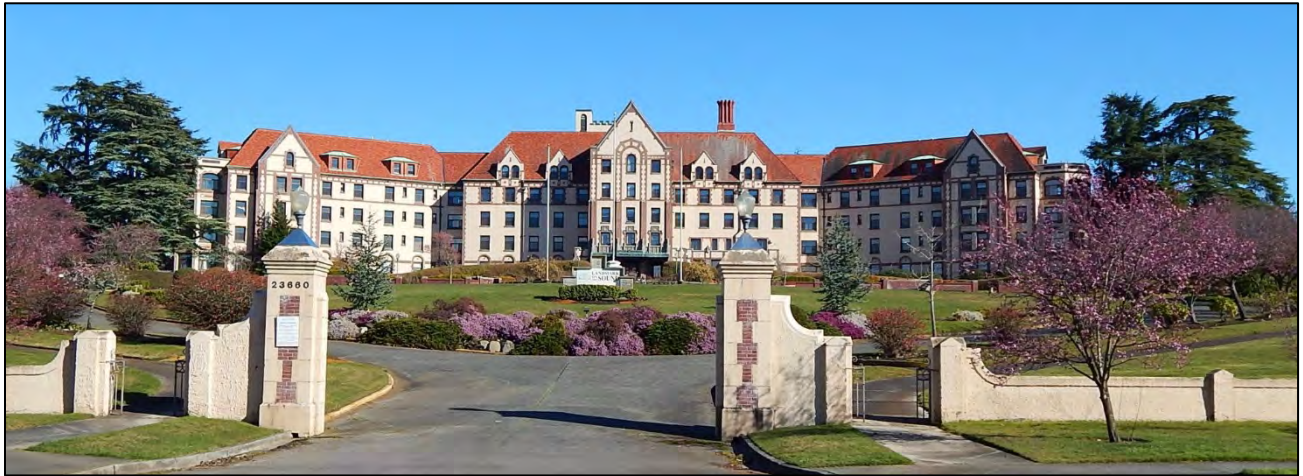
Fig. 1 – Main building, west elevation from front gates, view in 2018. (Ron Clausen Wikimedia Commons)
