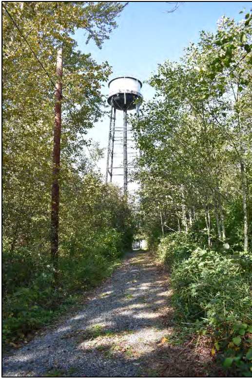
Fig. 97 – Water Tower (built 1926).
