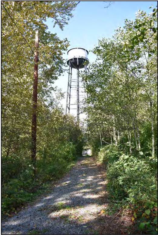
Fig. 38 – Water Tower (built 1926).
