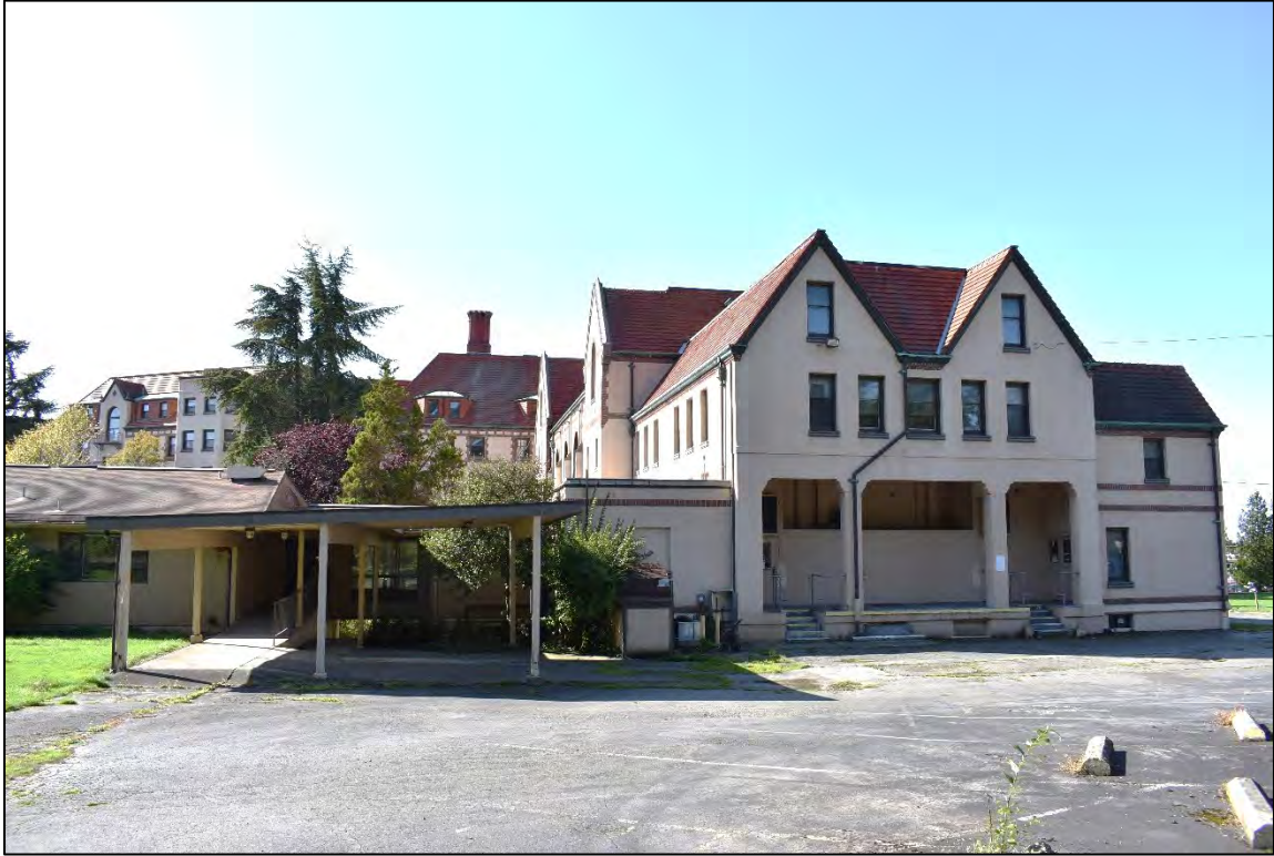
Fig. 16 – Main building, south and east elevations, rear service wing, showing loading dock and Infirmary Wing.
