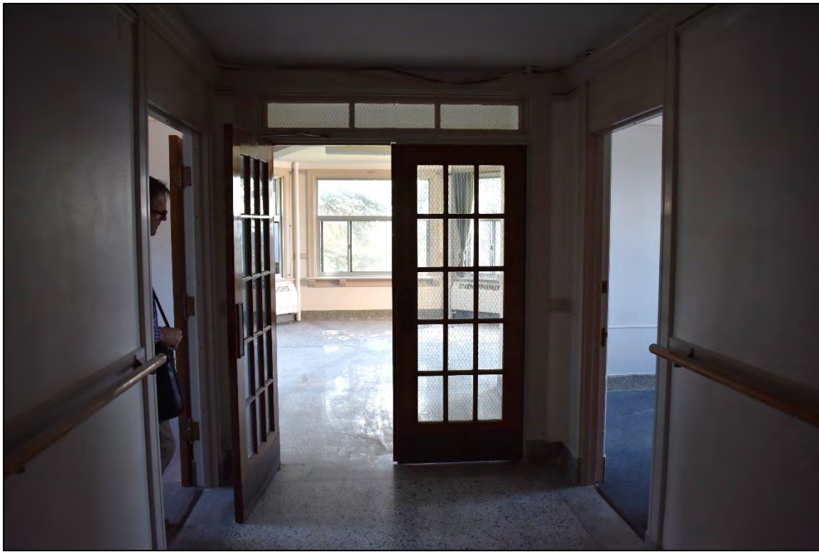
Fig. 81 – Main Building, interior, upper floor, typical solarium at end of residential corridor.
