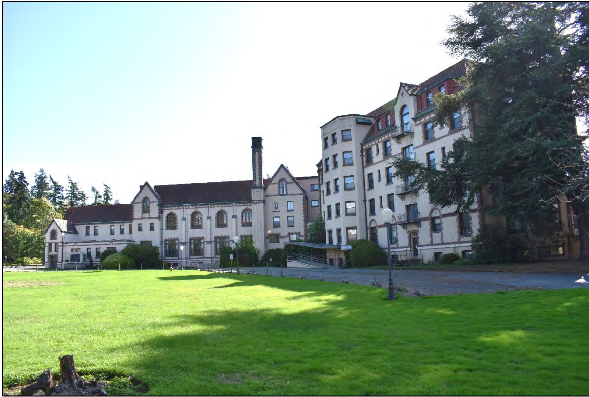
Fig. 12 – Main building, view south to east and north elevations.
