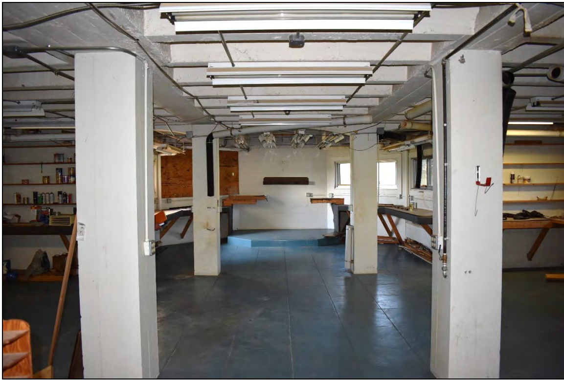
Fig. 89 – Main Building, interior, basement, typical room.
