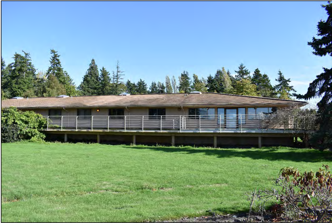
Fig. 32 – Infirmary Wing, southwest arm (built 1987), west elevation.
