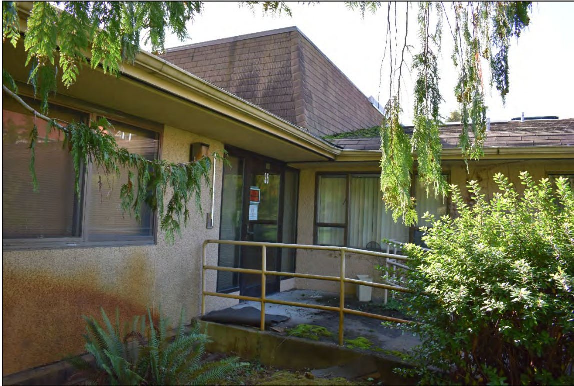
Fig. 22 – Infirmary Wing, juncture of east arm (at left, built 1987) and north arm (at right, built 1966).
