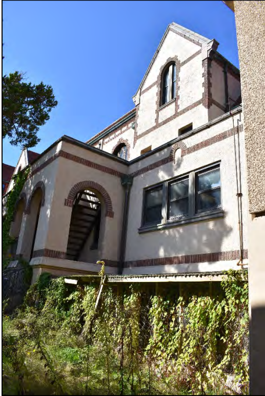
Fig. 17 – Main building, south elevation facing Infirmary Wing courtyard.
