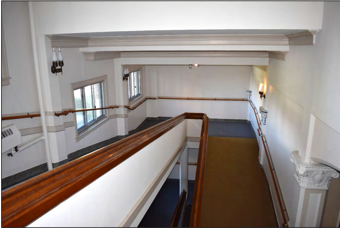
Fig. 60 – Main Building, interior, second floor, main circulation ramps.
