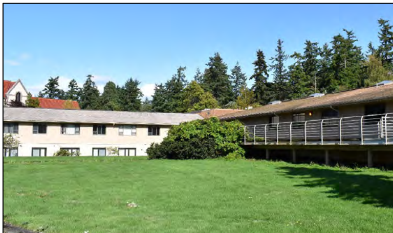
View from southwest yard: 1966 Infirmary Wing on left, 1987 addition on right.
