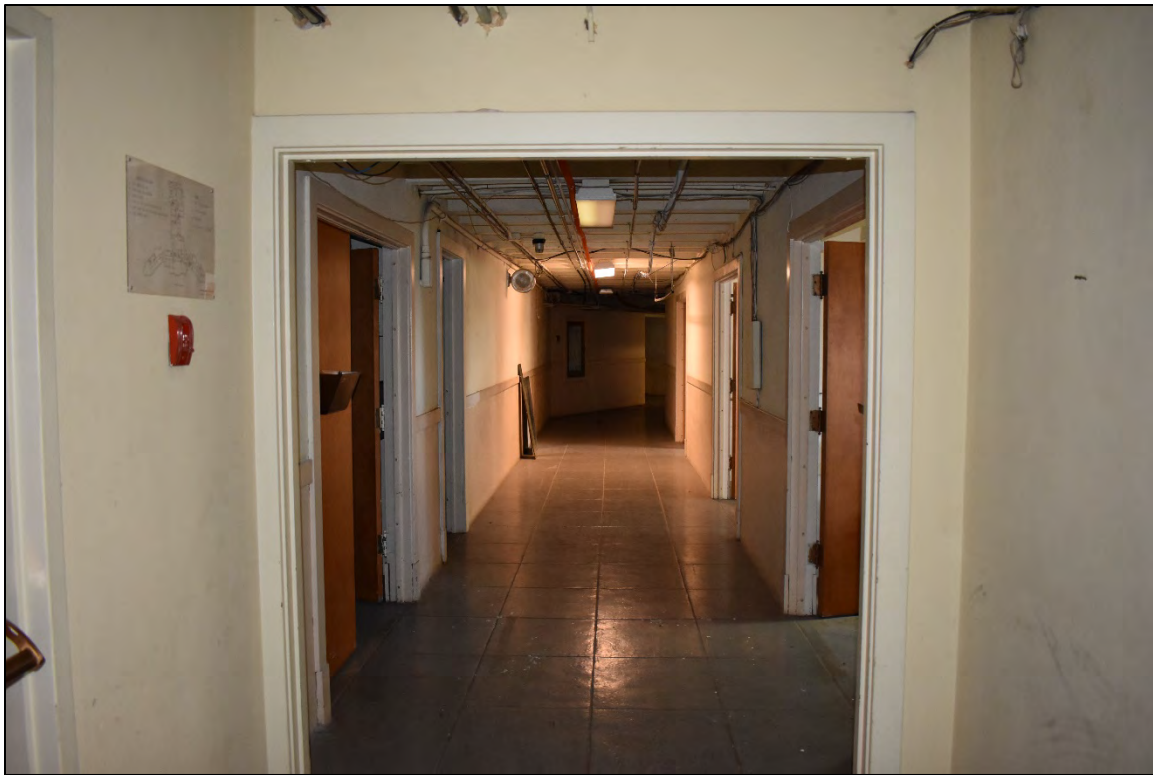
Fig. 87 – Main Building, interior, basement, typical corridor.
