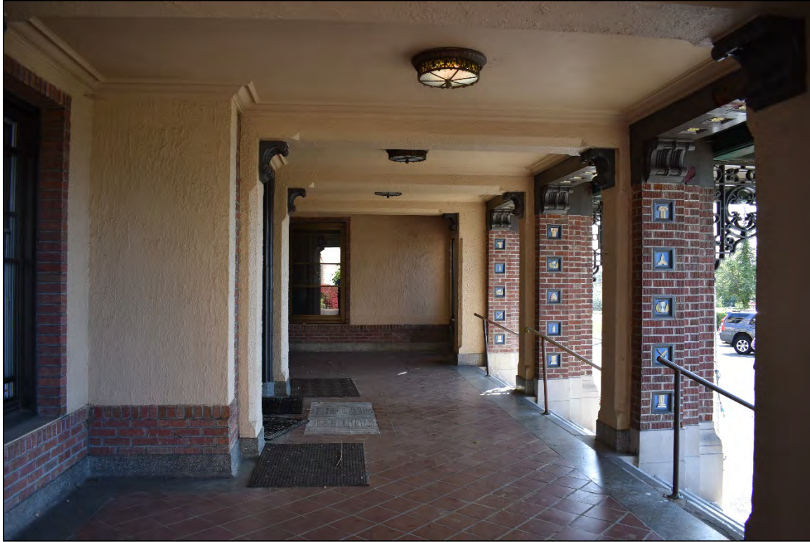
Fig. 8 – Main building, west elevation, main entrance porch.
