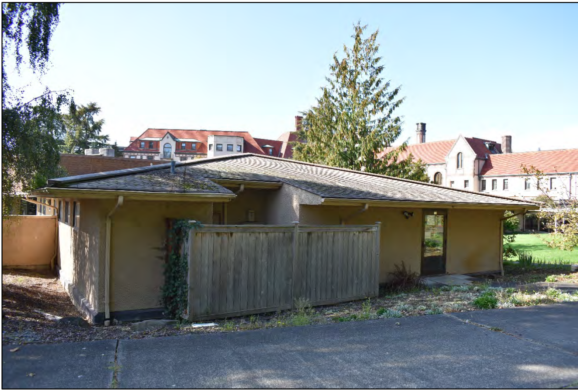
Fig. 23 – Infirmary Wing, east elevation of east arm (built 1987).
