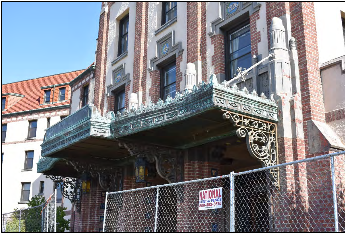
Fig. 7 – Main building, west elevation, main entrance marquee.
