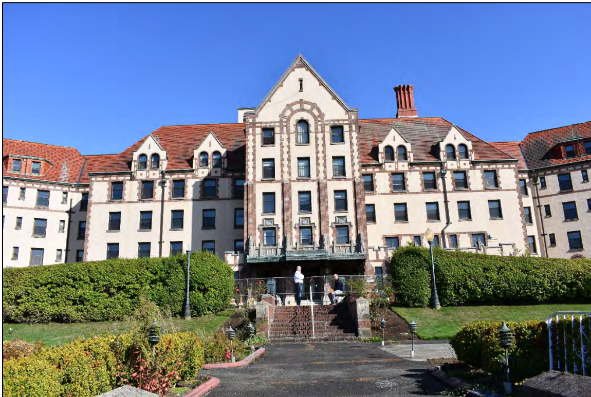
Fig. 2 – Main building, west elevation.
