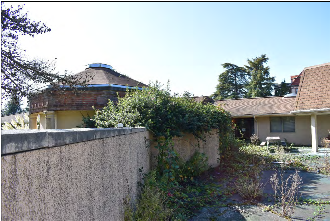
Fig. 27 – Infirmary Wing, outdoor walled exercise area, view west towards building.
