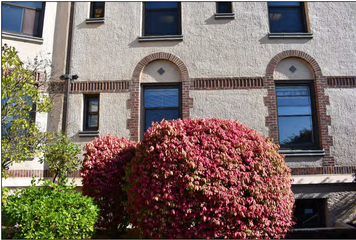
Fig. 5 – Main building, west elevation of central portion, detail of wall.
