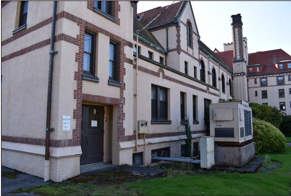
Fig. 14 – Main building, north elevation.
