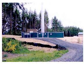
Ground mounted facilities shall provide a shelter and screened enclosure to minimize visual impact.
