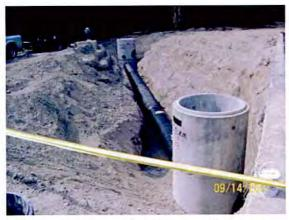
Stormwater systems should be installed at appropriate depth for future development of undeveloped portions of the business park.
