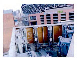
Screening of roof-mounted antennas, and equipment should be integrated into the design of the building
