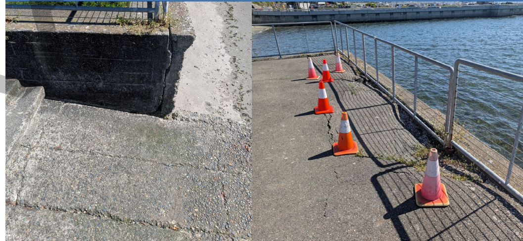
Bulkhead Failure
