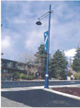
Parking lot lighting
