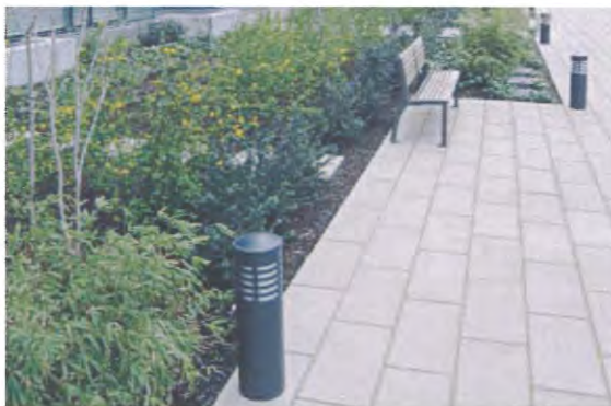
Use of bollards as pedestrian pathway lighting
