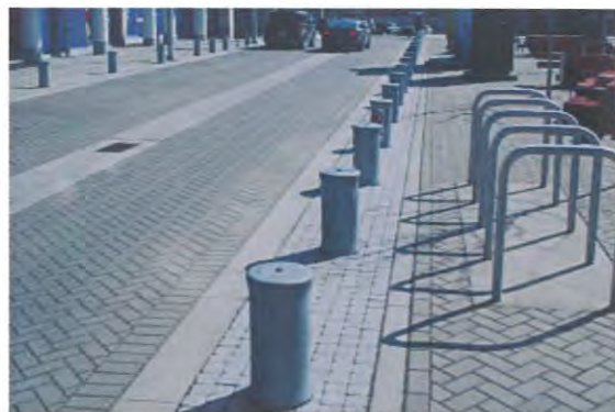
Bollards help define pedestrian and vehicular traffic
