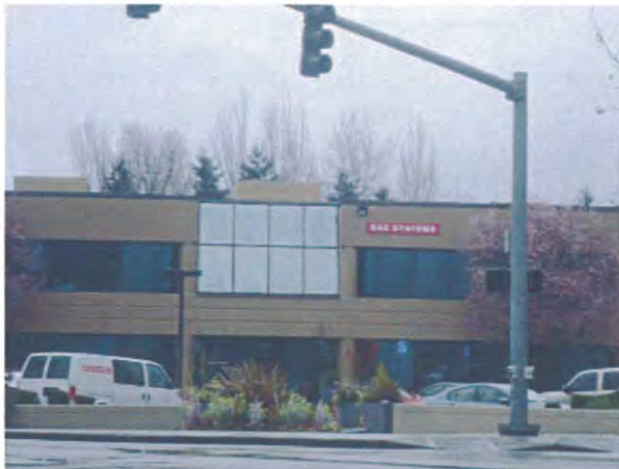
Building modulation and changes in window types help to create visual interest.
