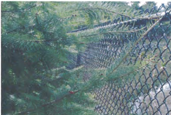
Use of black vinyl coated fencing at site perimeter
