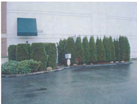
Use of landscaping and fencing to screen trash and recycling areas.
