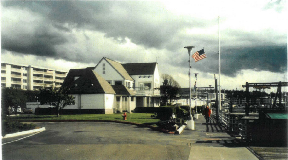
Figure 6-1. Marina Office Building
