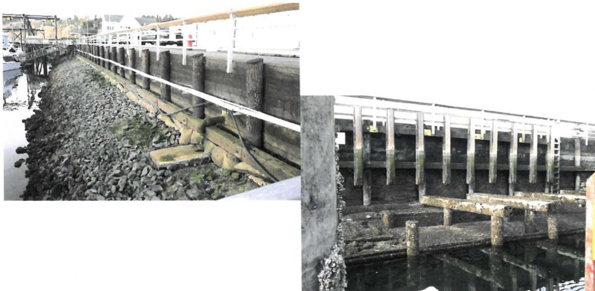
Figure 2-2. Timber Pile Bulkhead
