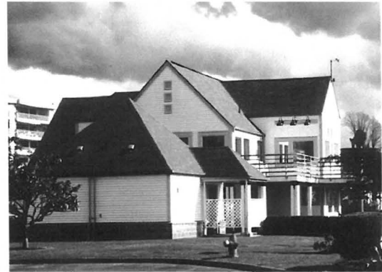
Figure 5-1. Marina Office Building
