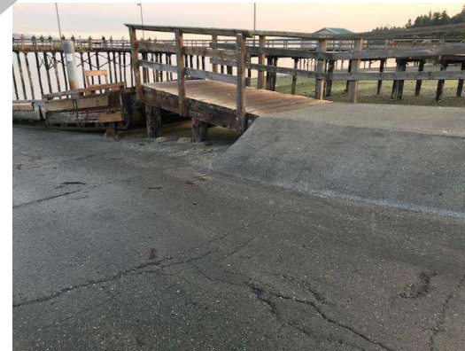
Des Moines City of; Redondo Boarding Floats Upgrades Phase 2 (#24-2501) Attachment #641607, Concrete & Timber Approach to be replaced.jpg
