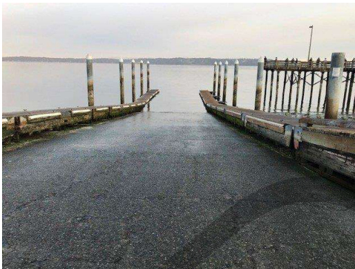
Des Moines City of; Redondo Boarding Floats Upgrades Phase 2 (#24-2501) Attachment #641605, North & South float Strings.jpg
