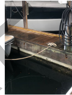
Photo 11. Timber Float with Unencased Flotation
