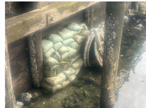
Photo 11. Timber Float with Unencased Flotation
