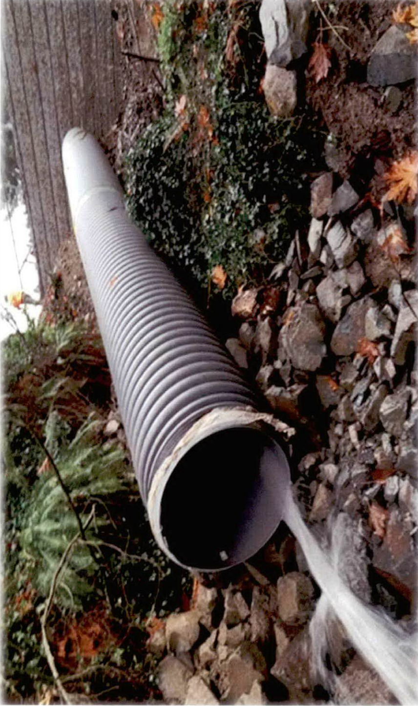
S. 251st Street Storm Outfall
