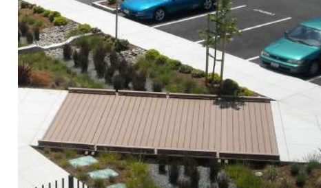
Pedestrian bridge over bioswale
