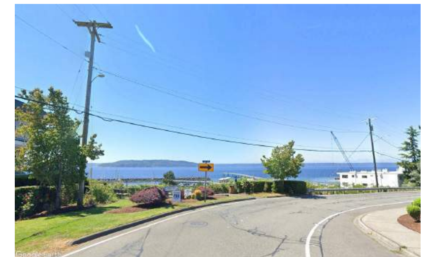
Overhead utility lines at Overlook I Park
