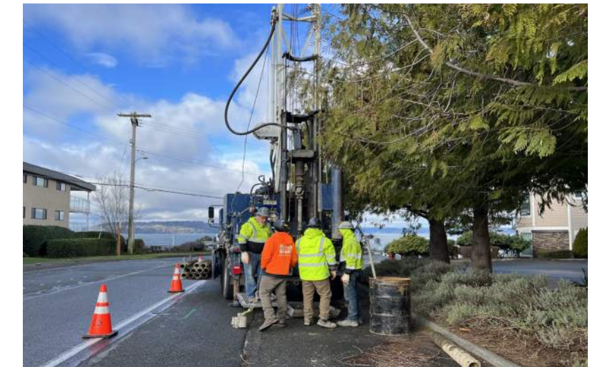
Geotechnical boring along South 223rd Street
