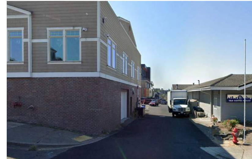
Utility undergrounding completed in Des Moines Theater alley at S 223rd St.
