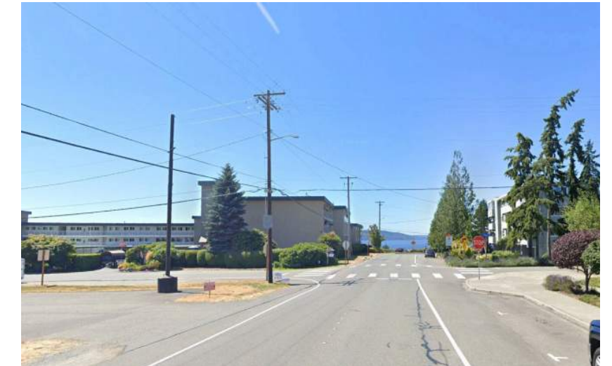
Overhead utility lines at S 223rd St and 6th Ave S intersection
