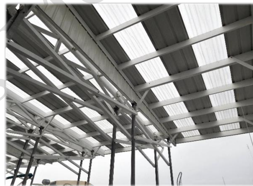
Figure 4-3. Light-Penetrating Covered Moorage
