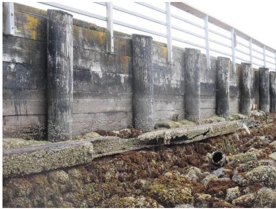
Figure 2-13. Existing North Timber Pile Bulkhead
