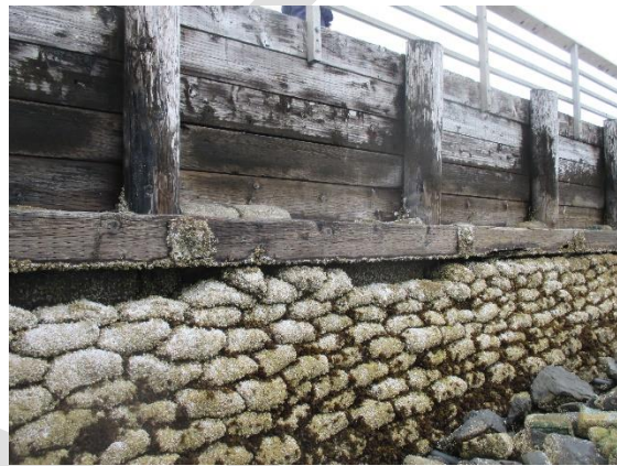
Figure 2-14. Existing West Timber Pile Bulkhead
