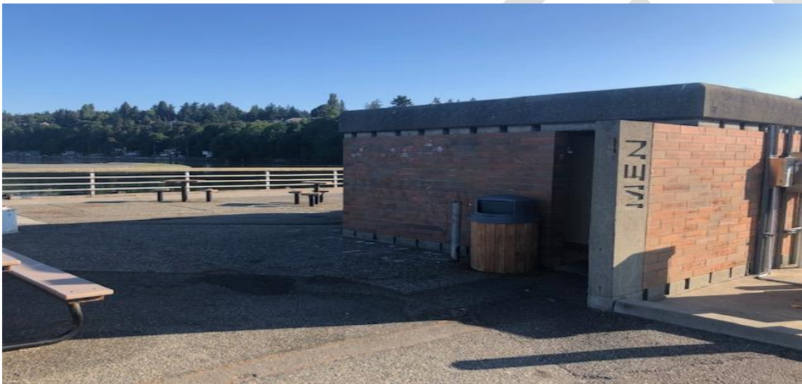
Figure 2-16. Public Restroom in the Waterfront Zone
