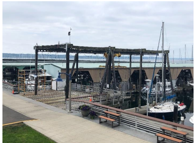
Figure 2-10. Dry Shed Launcher
