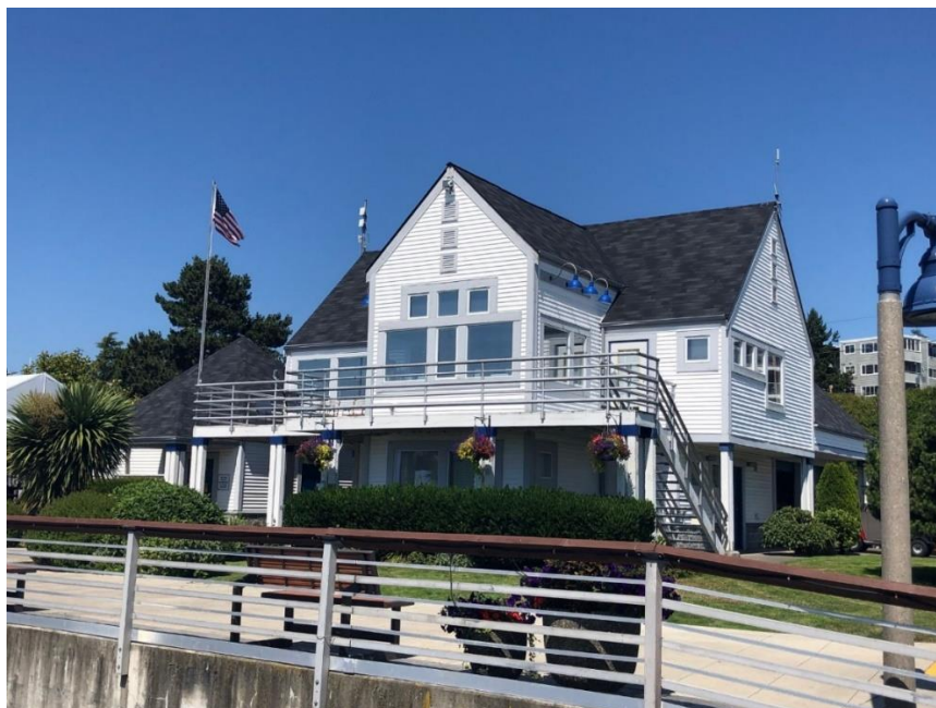
Figure 5-1. Marina Office Building July 2021
